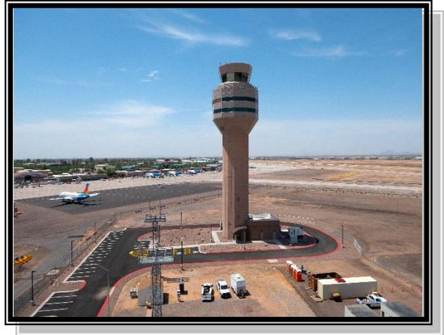
**Construction Method:** Precast Shaft / Steel Super Structure
