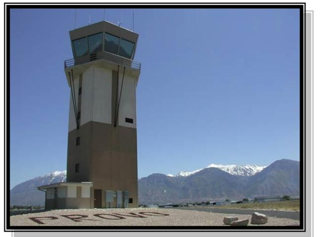
**Construction Method:** Precast concrete panels (Shaft) and Structural Steel Cab
