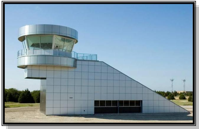
**Construction Method:** Steel w/ ReynoBond Panel System Cladding –Structural Steel Cab
