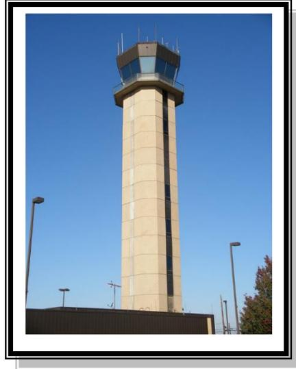
**Construction Method:** Structural Precast Concrete Shaft; Steel Frame Cab
