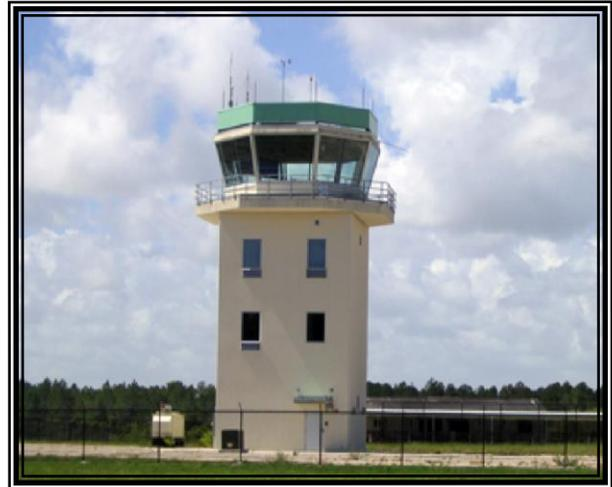
**Construction Method:** Site Cast, Concrete Panels - Shaft and Structural Steel Cab
