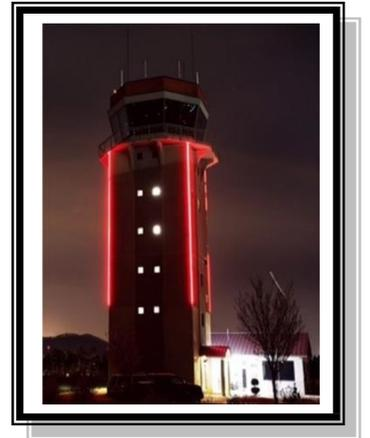
**Construction Method:** Structural Precast Concrete Shaft; Steel Frame Cab
