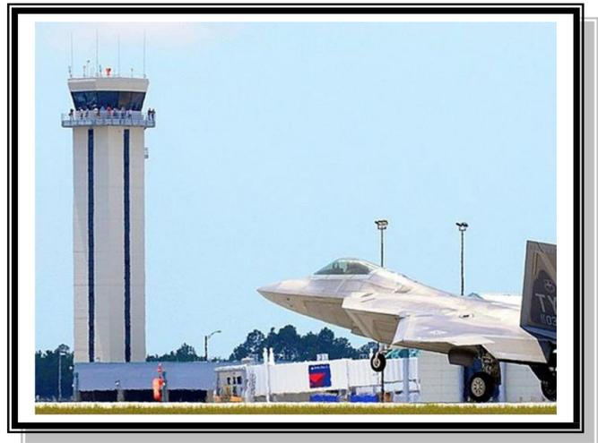
**Construction Method:** Poured-in-place Concrete Shaft (9 floors); Steel Frame Cab
