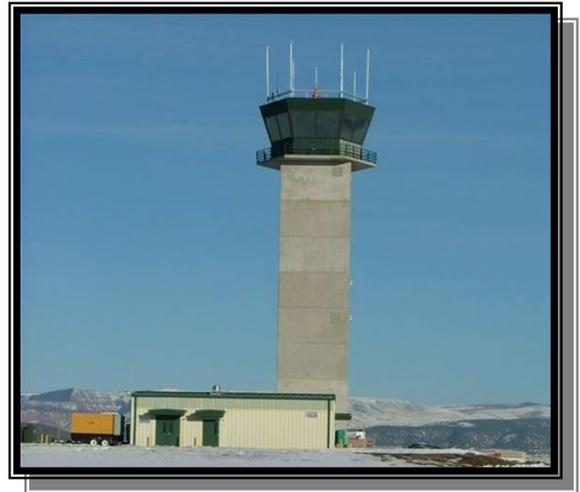
**Construction Method:** Precast Concrete panels with Structural Steel Cab
