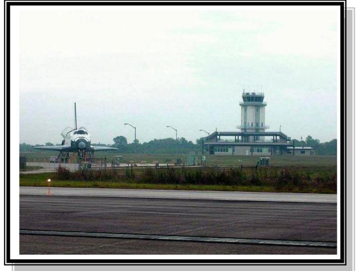
**Construction Method:** Precast Concrete Panels, Structural Steel Cab
