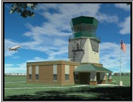
**Construction Method:** Structural Steel with combination Brick and Precast Concrete Panel Cladding
